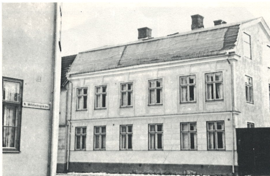
Nr: 13, kv Reval
